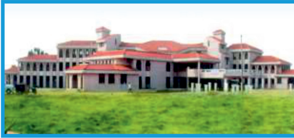
SDM College of Ayurveda and Hospital, Hassan
