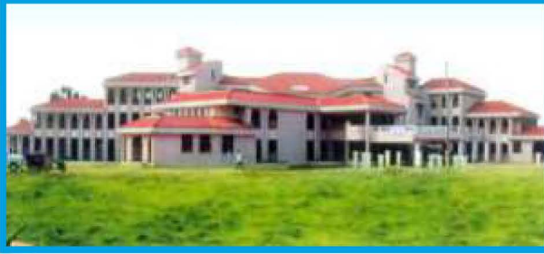
SDM College of Ayurveda and Hospital, Hassan
