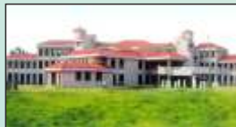
SDM College of Ayurveda and Hospital, Hassan
